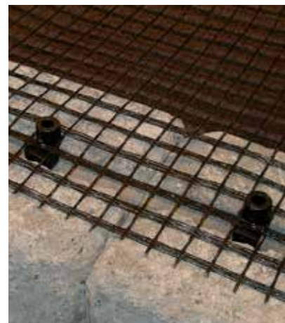
Fig 3. Fitting Bender Geonät (geogrid) to the first course. Secure the grid over the locking plugs. Have the plugs protruding from the third row of the grid. This is so that, without being visible, there is as much grid between the courses as possible. The grid is also then as secure as possible.
