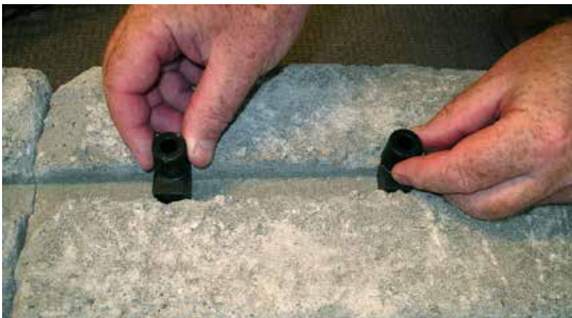
Fig 2. Fitting of Bender Låsplugg (locking plug), sloping wall. Fit two locking plugs per blockstone.
