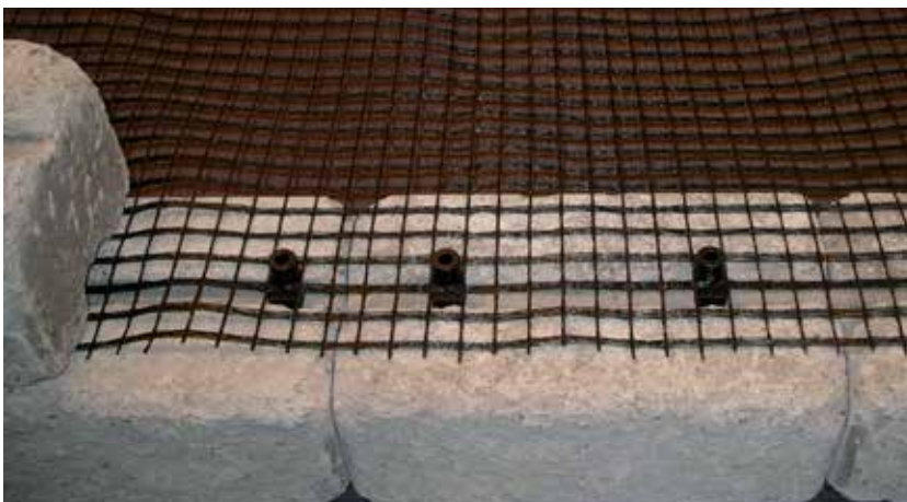
Fig 3. Fitting Bender Geonät (geogrid) to the first course. Secure the grid over the locking plugs. Have the plugs protruding from the third row of the grid. This is so that, without being visible, there is as much grid between the courses as possible. The grid is also then as secure as possible.
